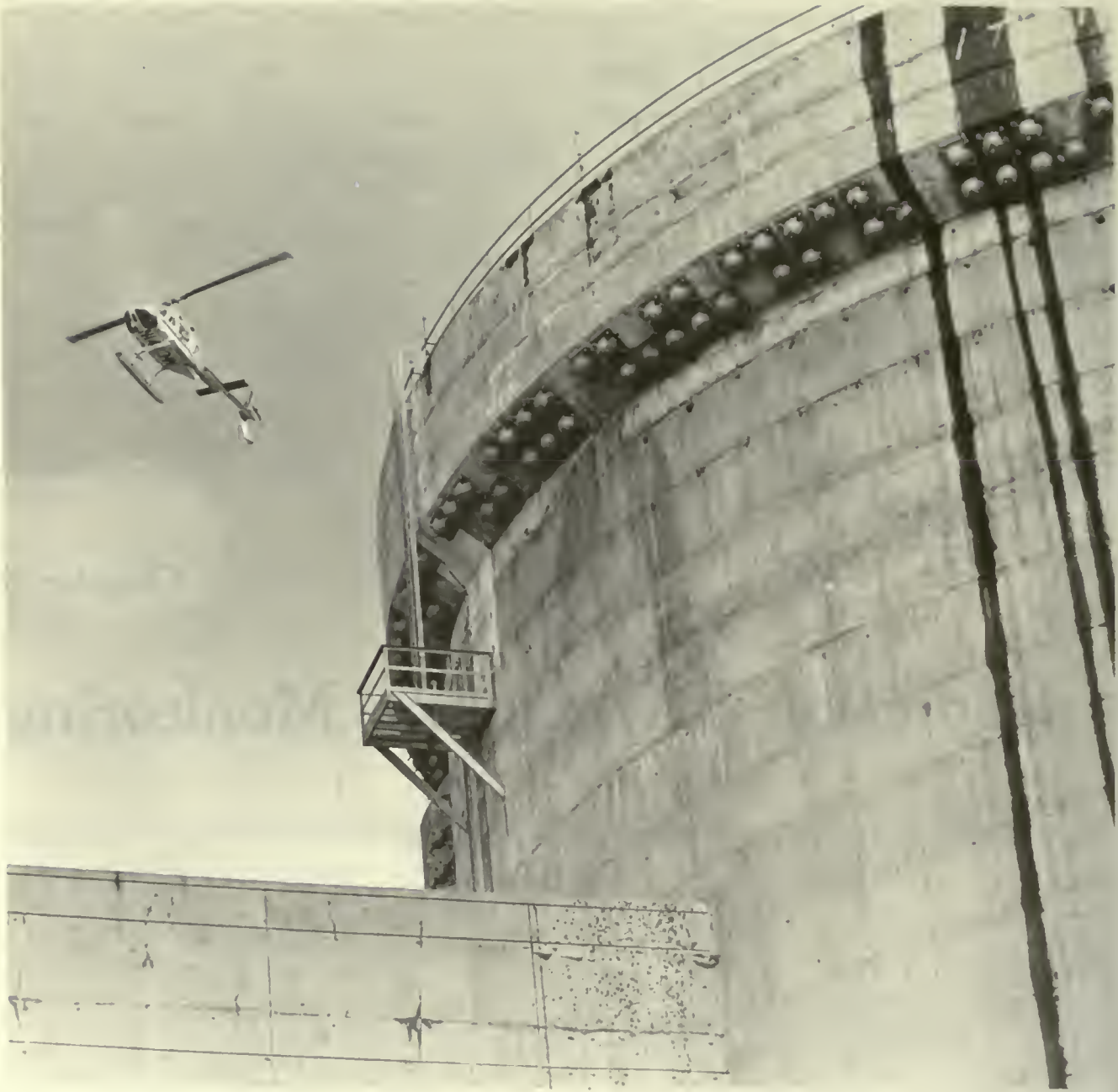
Helicopter monitoring radiation releases during March 28, 1979 accident
