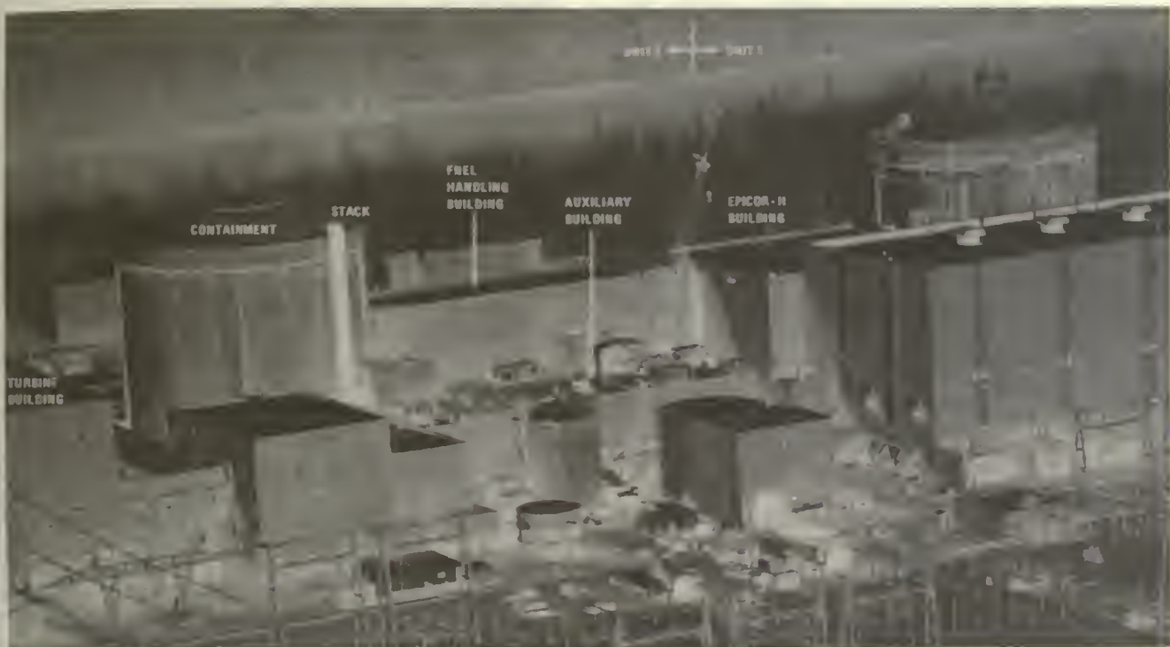
Major buildings of Unit 2, Three Mile Island Nuclear Station, including the Epicor-II
