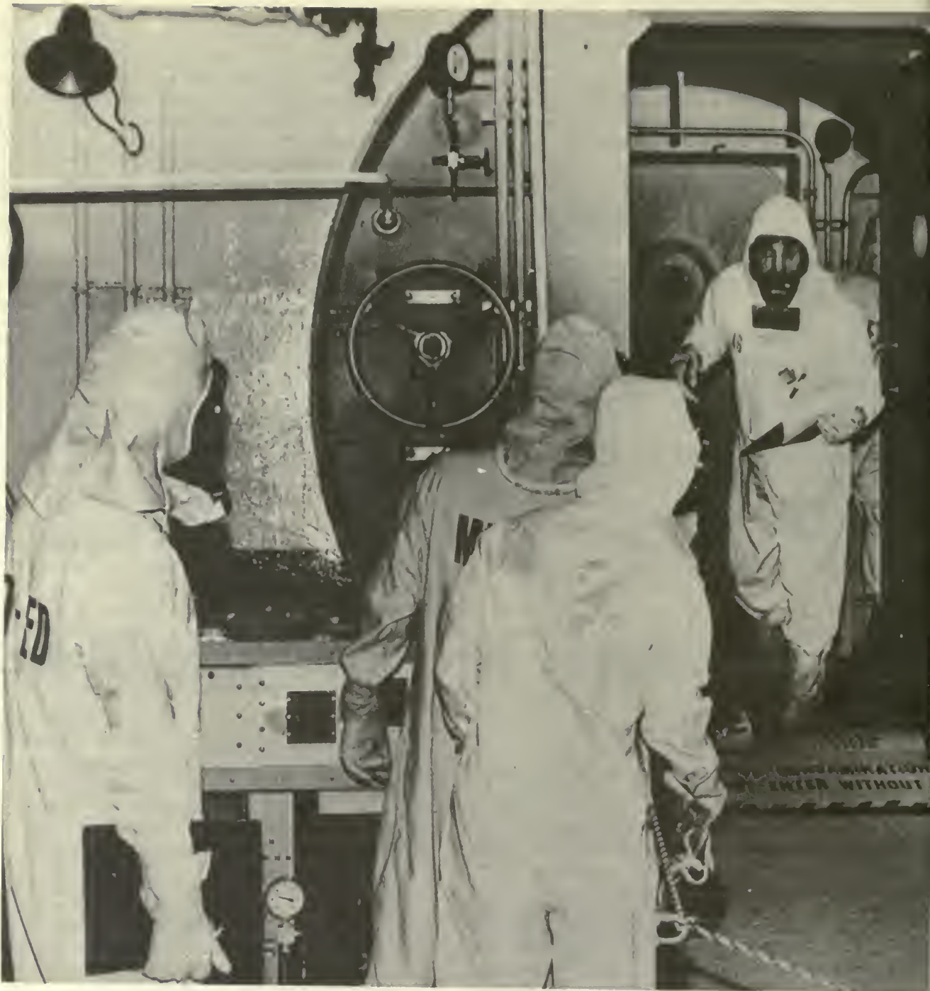
Cleanup workers at Three Mile Island gain access for the first time to the airlock leading to the containment. Beyond the second door are the damaged reactor and other major components of the plant's primary system
