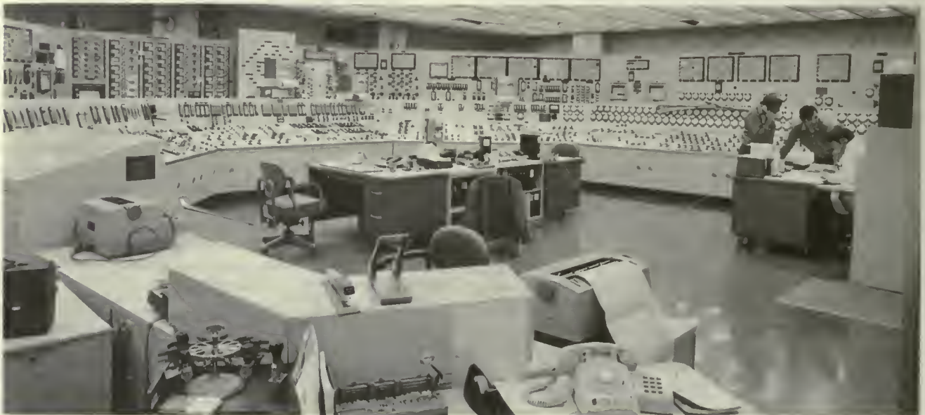
The control room at Three Mile Island, Unit 2
