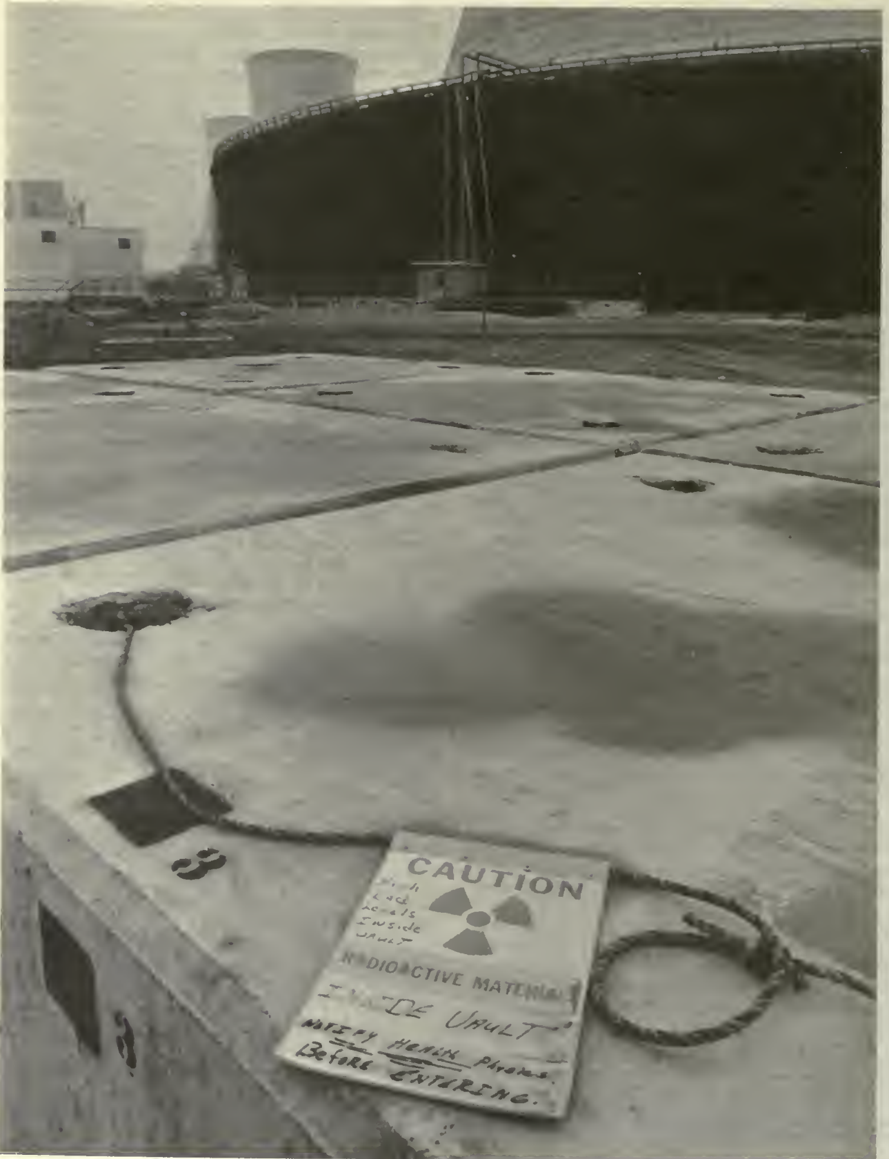
Storage vaults for radioactive wastes resulting from cleanup
